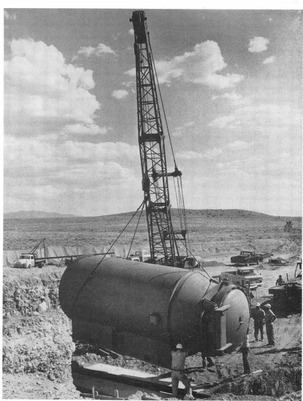
EASY DOES IT - A 37,000-lb. steel firing chamber in velop explosive-actuated power supplies. High speed Coyote Test Field will be part of a new facility to decameras, protected by heavy glass, will record results.
